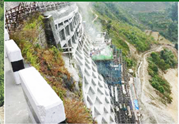
Ground anchor works
