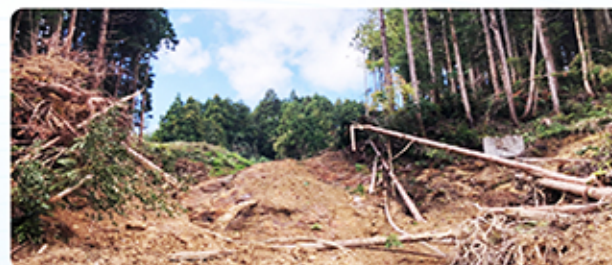
Collapsed Access Road
