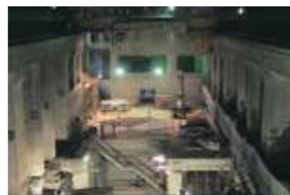
Powerhouse at Musi Project, Indonesia
