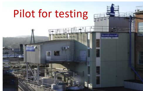
The SEKAB plant Sweden
