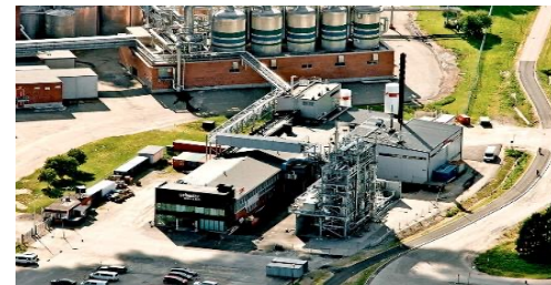
LTU Green Fuels' plant in Piteå
