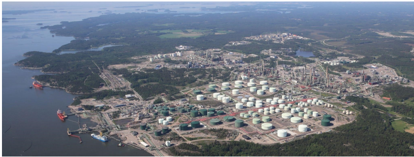
NESTE's HVO biorefinery, Poorvo, Finland
