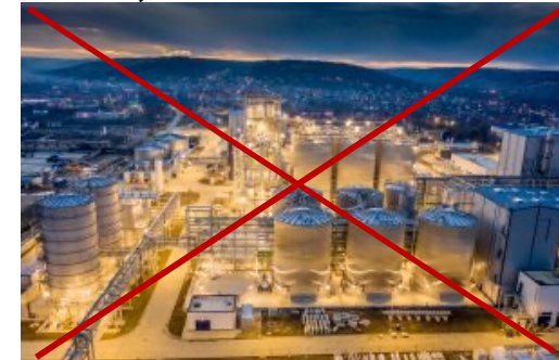
Clariant's cellulosic ethanol plant Craiova, Romania
