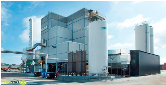
BTG's Empyro pyrolysis plant
