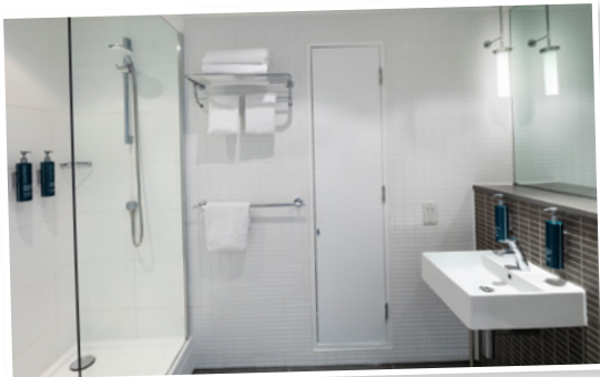
Refurbished bathrooms at DoubleTree By Hilton Leeds with bulk amenities dispensers and water-saving showerheads and taps
