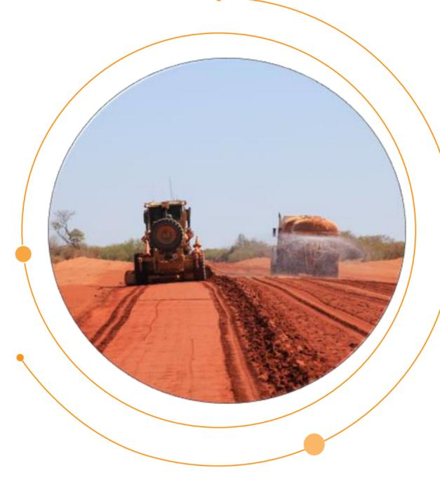
Polycom is a road base materials stabilisation agent. When mixed with the water on site it delivers a longer lasting running surface. Roads treated with PolyCom have lasted up to four times longer before requiring the regular maintenance programs as scheduled. This contributes significantly to long term asset management plans.
