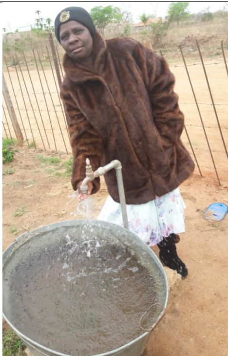
Happy water consumer in Matsikitsane village water reticulation project designed by Dalimede Projects
