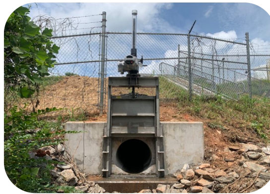
Retrofit of adaptive outlet structure
