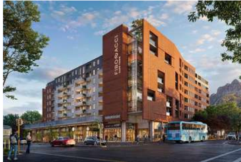
A new mixed use development along Sea Point Main Road
