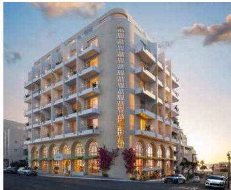
A new mixed use development along Sea Point Main Road
