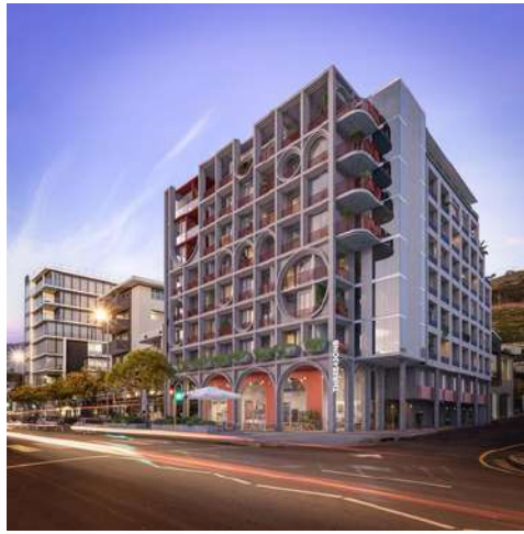
A beautiful new mixed use development along Sea Point Main Road by BLOK and 255 Architects
