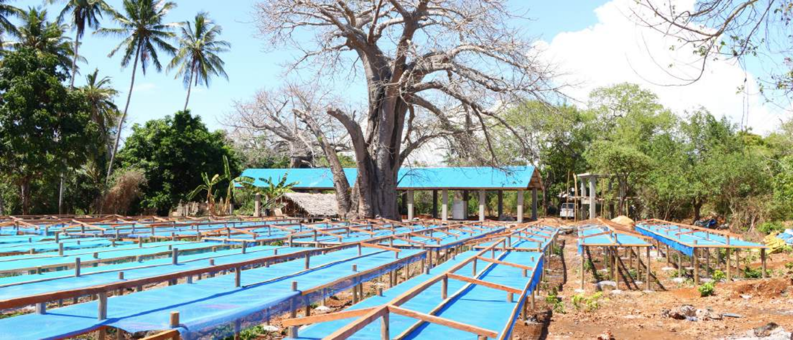
The constructed Kibuyuni dagaa processing area and drying racks.
