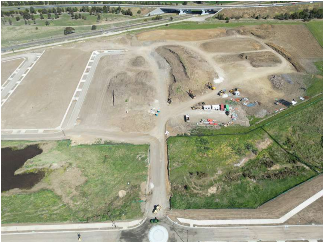
Figure29: Image of a construction site
