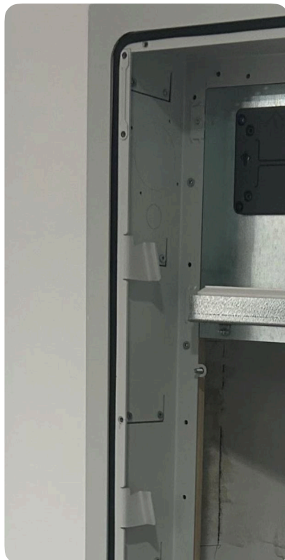
Figure 10: Detailed picture of the flaps and the amount of screws required to secure the system.
