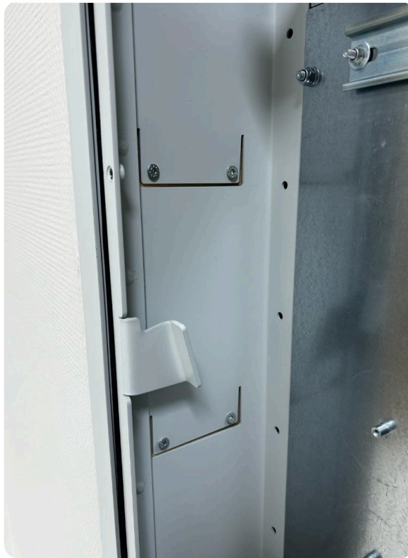
Figure 11: Detailed picture of the flaps and the amount of screws required to secure the system.
