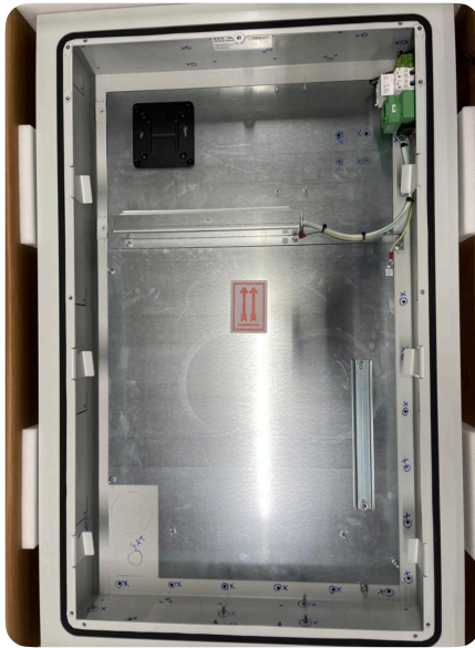
Figure 3: Mounting frame without cover plate.
