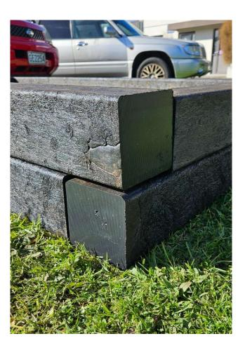
**3** - Measure 240mm from each end and mark with chalk, then 50mm diagonally from each corner and mark with chalk
