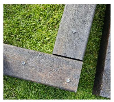
\*3a, 4a, 5a - For a custom box with joins along the sides/ends, measure, pre-drill and screw 100mm either side of each join
