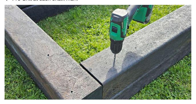
**5** - Then use the COUNTERSUNK screws to join these two layers. Keep checking alignment as you go. There will be a bit of movement
