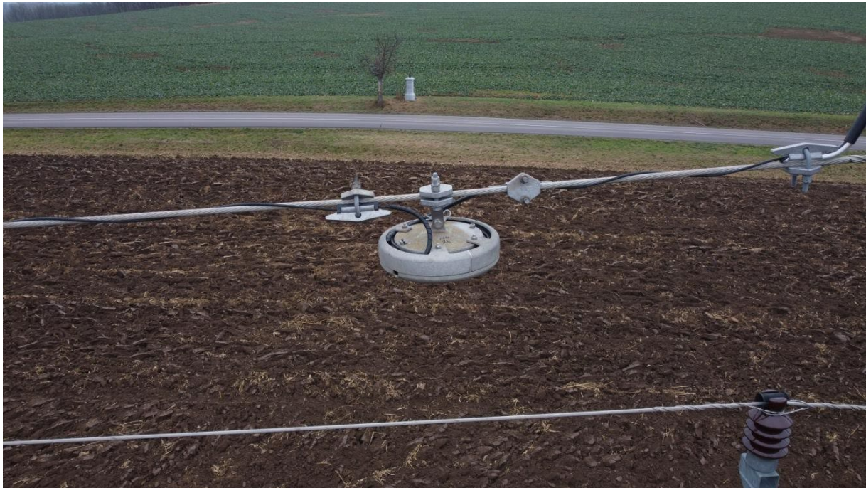
Fig. 7 – The disk connector attached directly to the conductor
