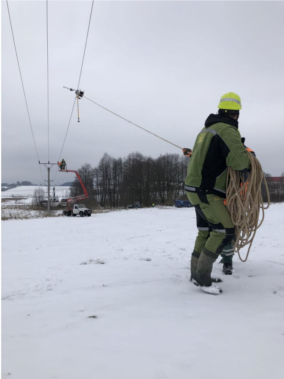
Fig. 4 – Installation of the optical cable
