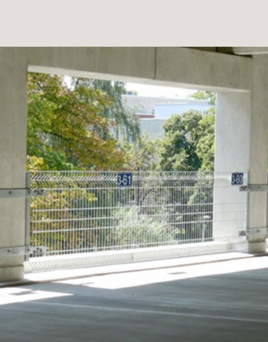
Supports impact loads up to 3.5 t and spanning up to 5.50 m without intermediate support
