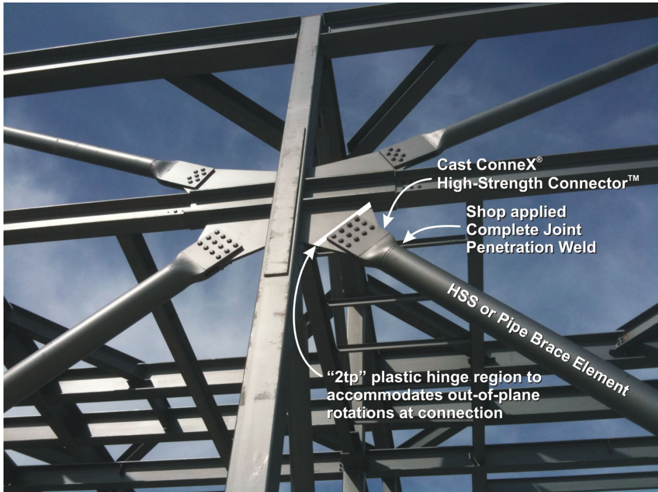
FIGURE 2—CAST CONNEX ® HIGH-STRENGTH CONNECTOR ™ SHOWN IN FIELD-BOLTED CONFIGURATION IN BRACED FRAME
