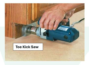
To dry cabinets in-place it will be necessary to remove the toe kicks to circulate air underneath the cabinets and possibly cut holes through drywall wall behind the cabinet, if the cabinets are installed on an interior wall, to access them from behind. Sometimes tenting hot, dry air from your dehumidifier will help raise vapor pressure differentials to dry and save the
