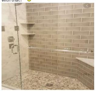
Ceramic tile is typically installed with wet mortar or thin set and grout. So, it is wet when it is first installed and stays wet for quite a while until it has a chance to acclimate.
