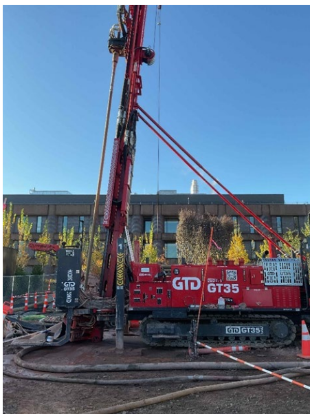
Figure 6-2. GTD GT 35 Drill Rig.
