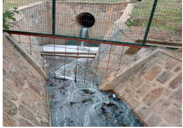
Industrial waste from special economic zone
