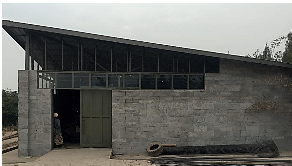
Photo 13: Photo of the front of the maintenance building.
