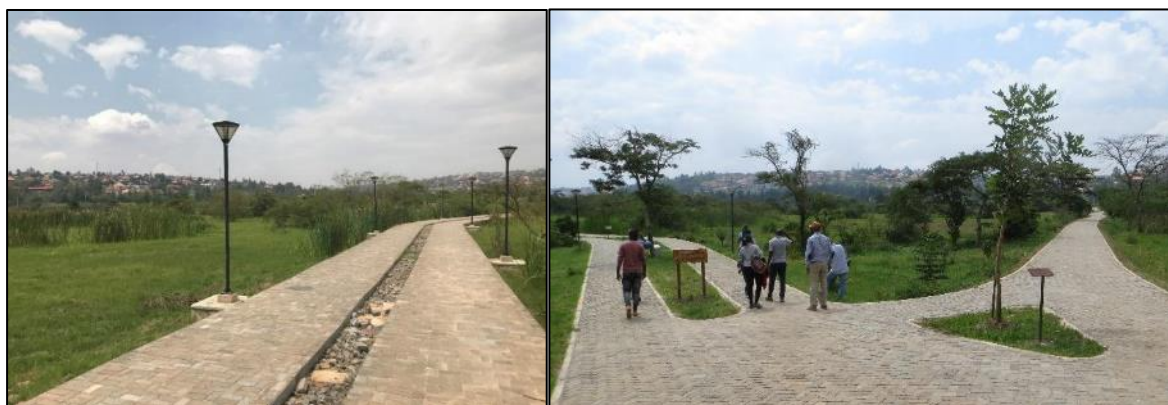
Photo 8: Bike paths (left) and pedestrian paths (right), and solar lighting along the path.
