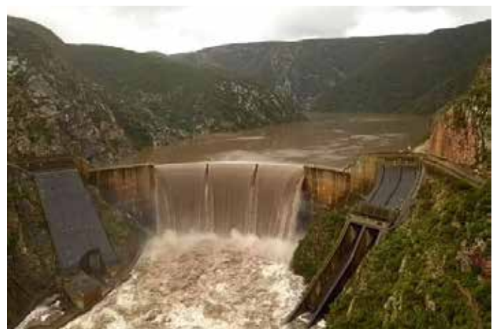
Overflowing Kouga Dam
