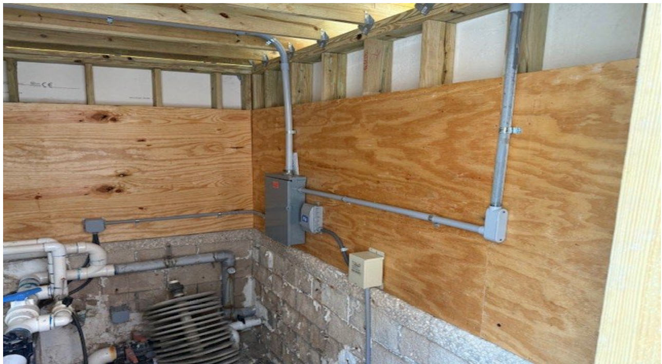
POOL EQUIPMENT HOUSE WITH RAISED ELECTRICAL
