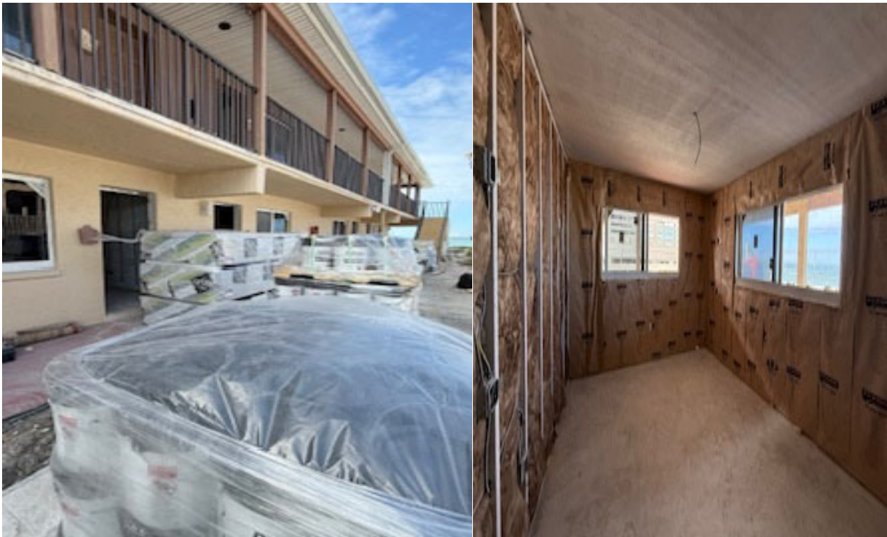
ARRIVAL OF SUPPLIES ON PROPERTY AND INSULATION INSTALL COMPLETED
