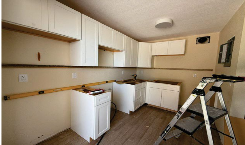
KITCHEN CABINET INSTALLATION ABOVE
