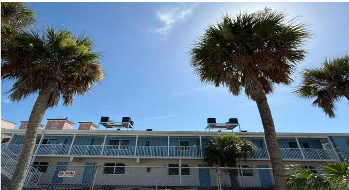
SHINGLES INSTALLED AND AC ROOF INSTALLATION
