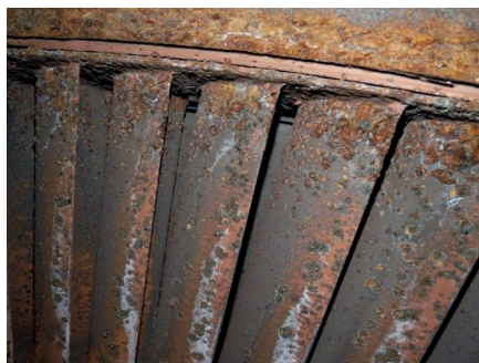
Figure 3. Corrosion of steam turbine blades.
