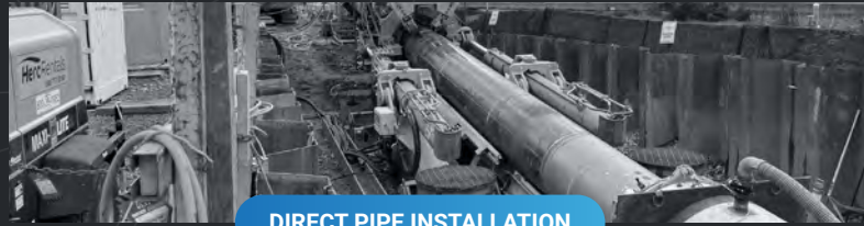
DIRECT PIPE INSTALLATION
