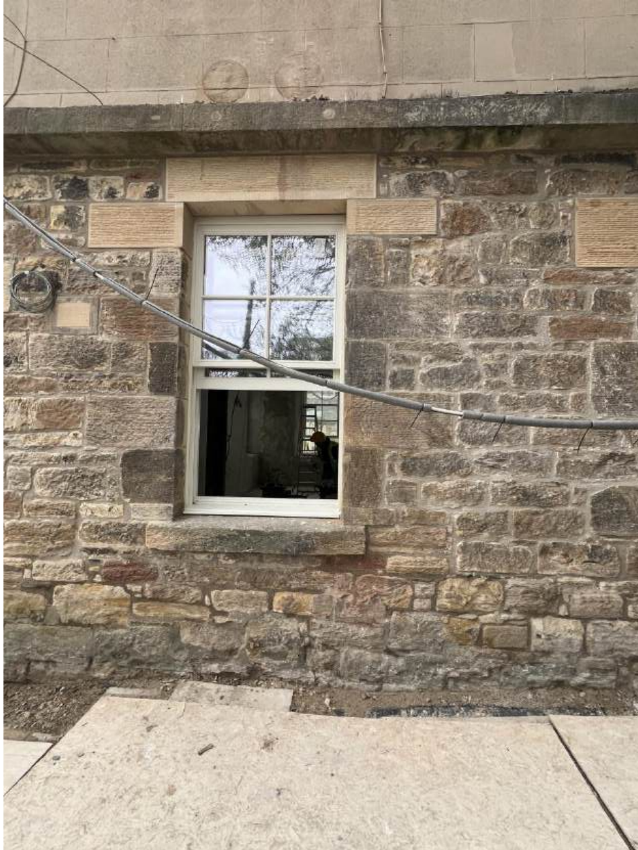
Window/IWI Detail – New S&C timber windows
