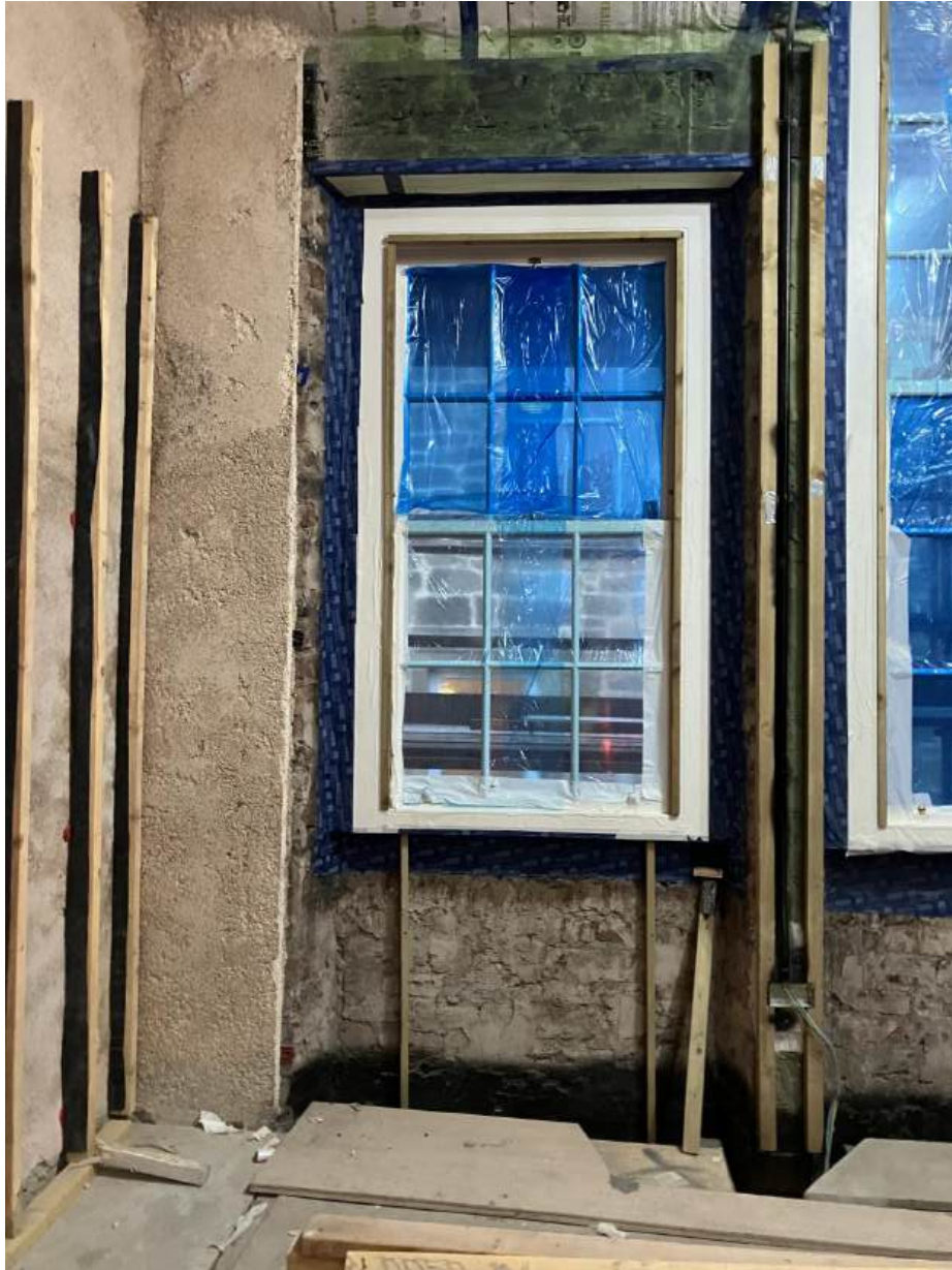
Window/IWI Detail – New S&C timber windows
