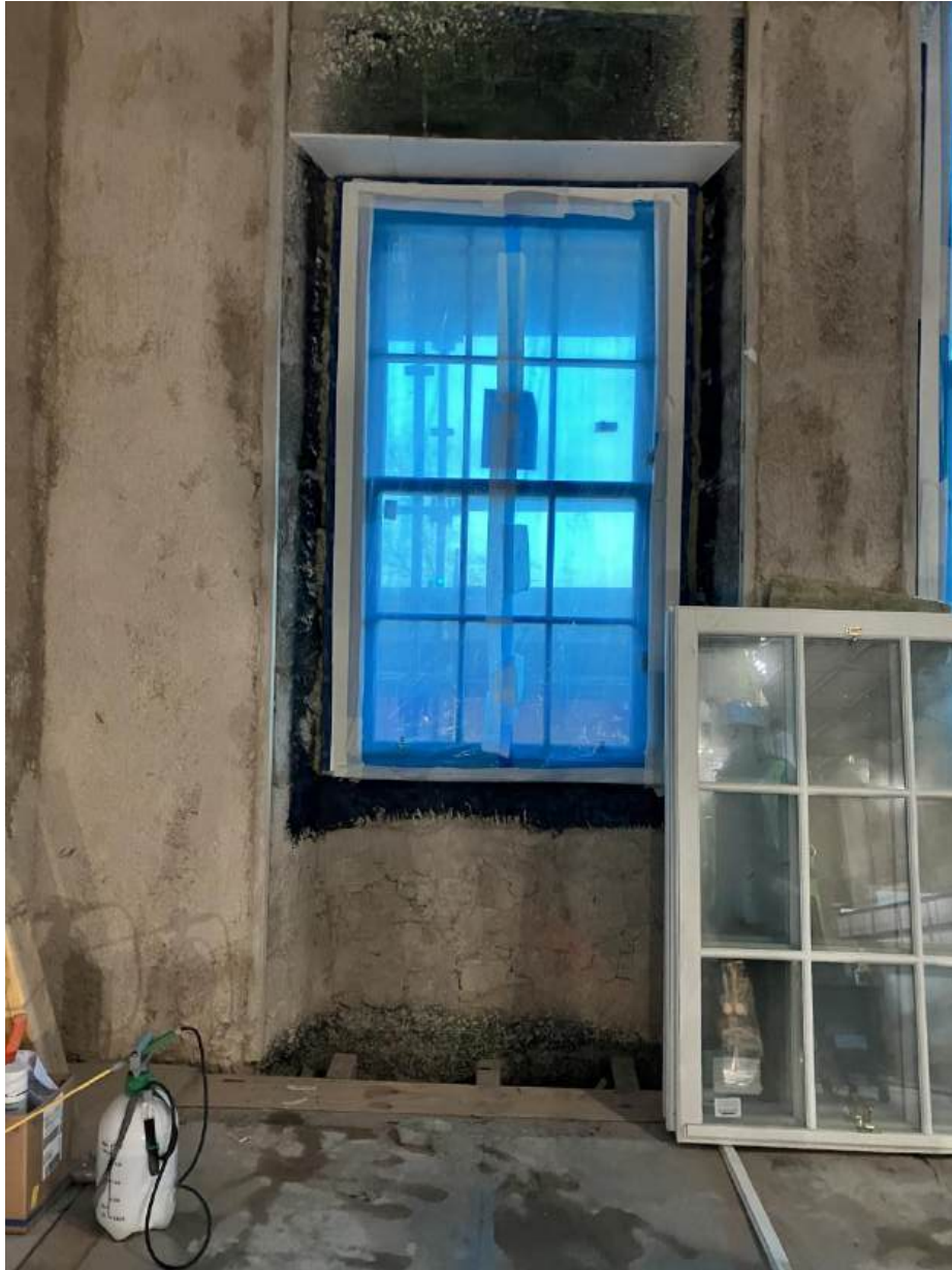
Window/IWI Detail – New S&C timber windows
