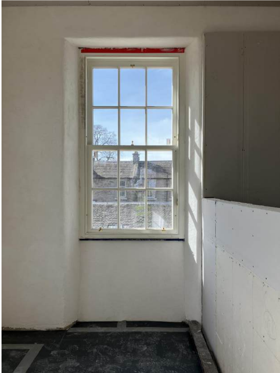
Window/IWI Detail – New S&C timber windows
