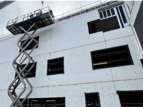
Karrier Panel Installation
