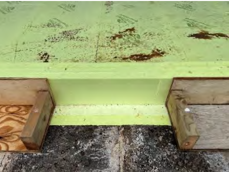
Underslab Insulation Installation
