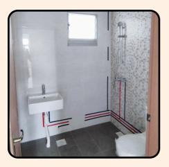
HDB doesn't allow for concealed pipings and hence, the default system is exposed plumbing, unless it's a BTO unit which originally comes with concealed pipings.
