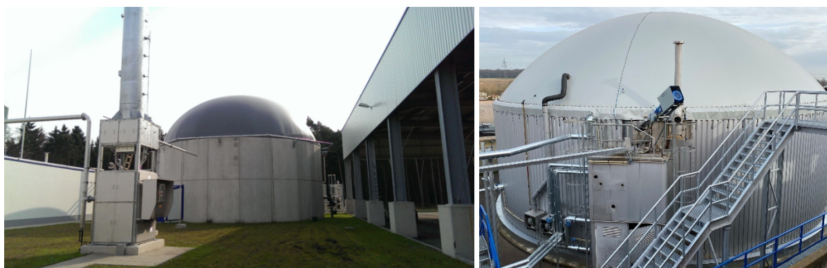
Gas flare and fermentation tank incl. gas holder (L) with mixer shown (R)
