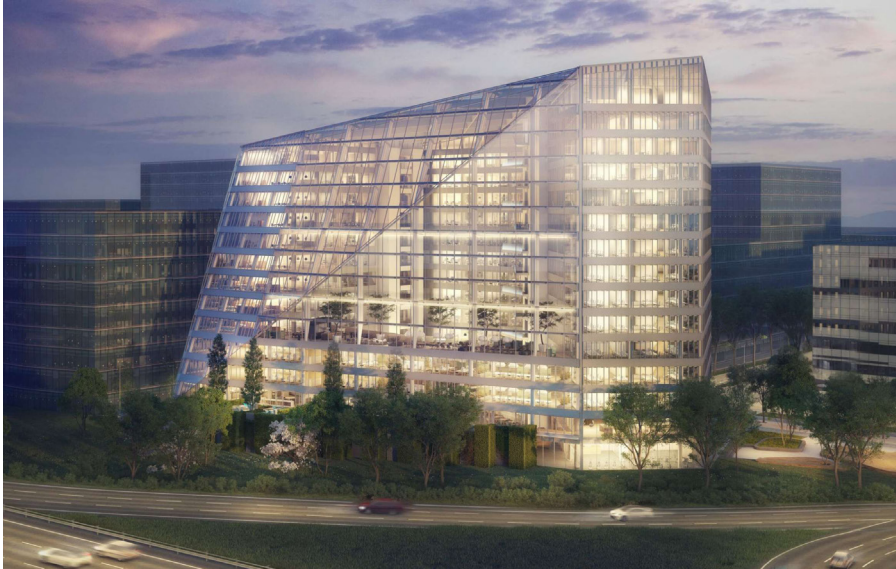
Mapiq helps The Edge in Amsterdam be one of the most innovative buildings in the world.
