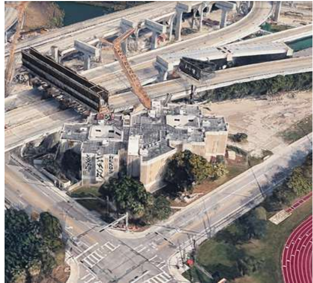
AERIAL VIEW SHOWCASING CURRENT CONDITIONS OF THE DETENTION CENTER
