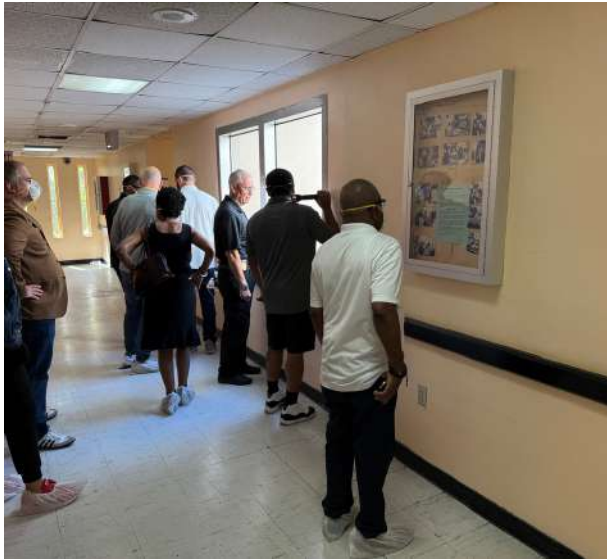
INTERIOR VIEW SHOWCASING CURRENT CONDITIONS OF THE DETENTION CENTER
