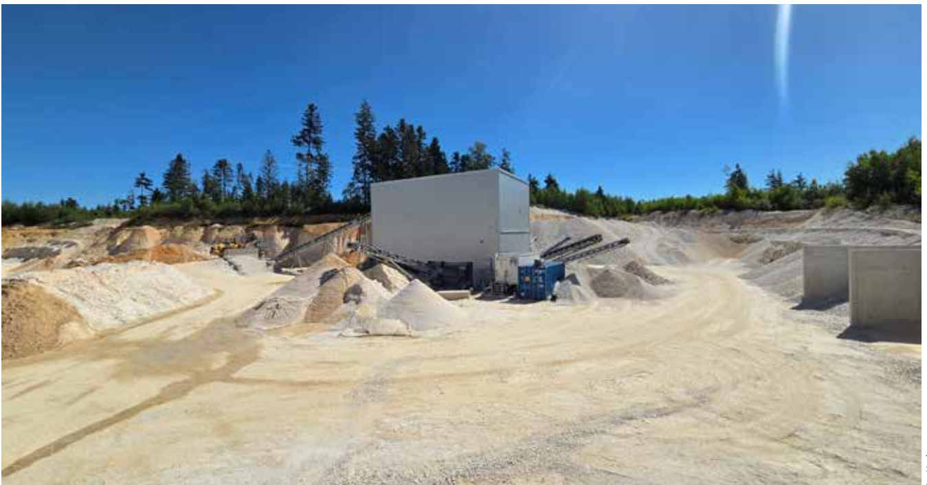
»1: State-of-the-art processing plant at the Freinberg open-pit mine in Upper Austria
