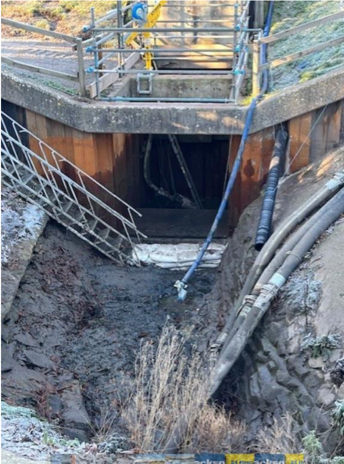
Lapperditch Piles Prepped for Over Plating
