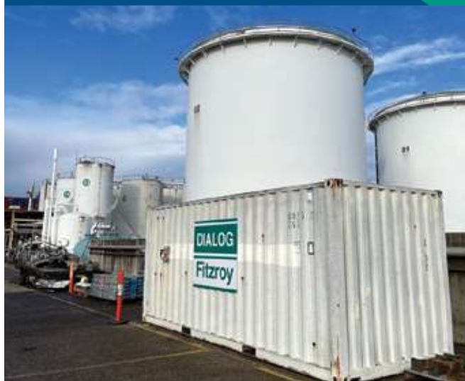
Tank inspection and maintenance for Quantem, Australia
