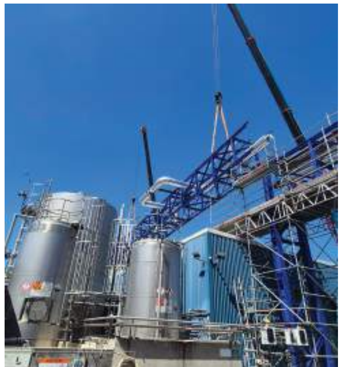
Fonterra Pipe bridge project Kakariki Whareroa New Zealand
