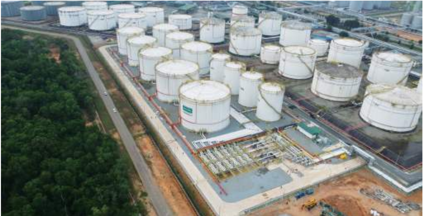
Phase 2 renewable fuel storage expansion at DIALOG Terminals Langsat 3
