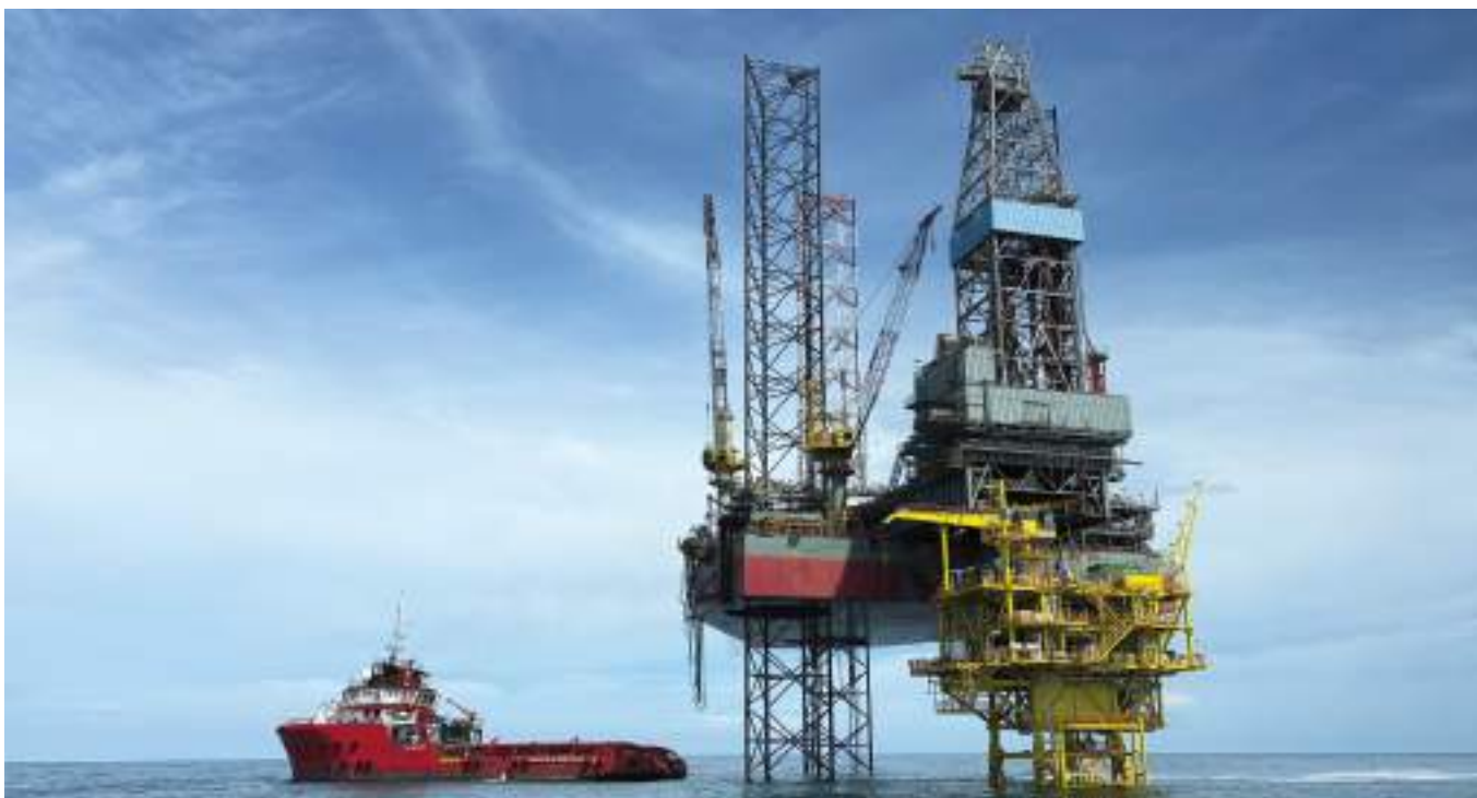
Drilling campaign at Salbiah wellhead platform offshore Miri, Sarawak
