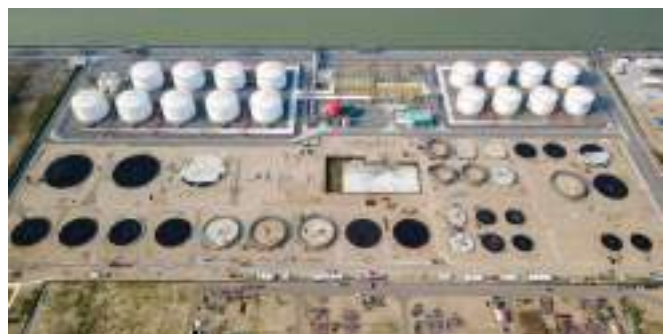
Construction site of the expansion of DIALOG Terminals Pengerang (5) Sdn. Bhd.
