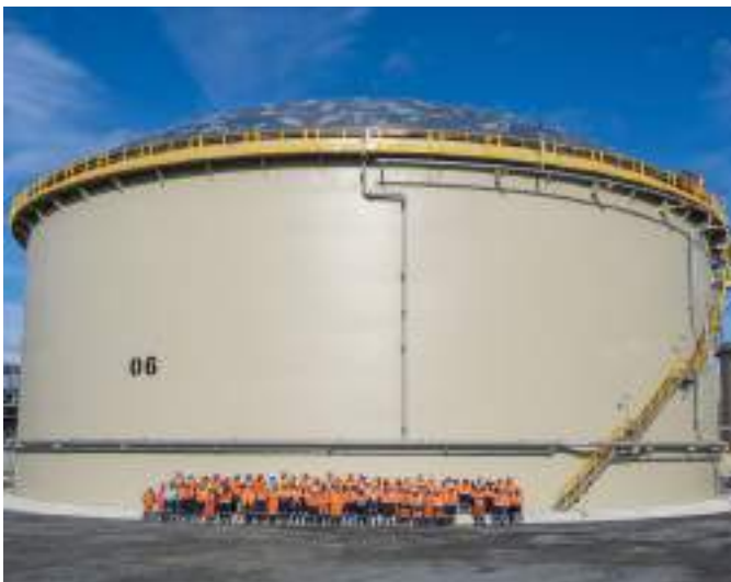
Channel Infrastructure T06 Conversion Project, Marsden Point, New Zealand
