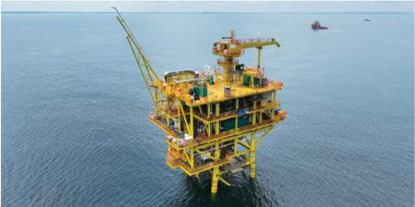
Installation of Salbiah wellhead platform offshore Miri, Sarawak
