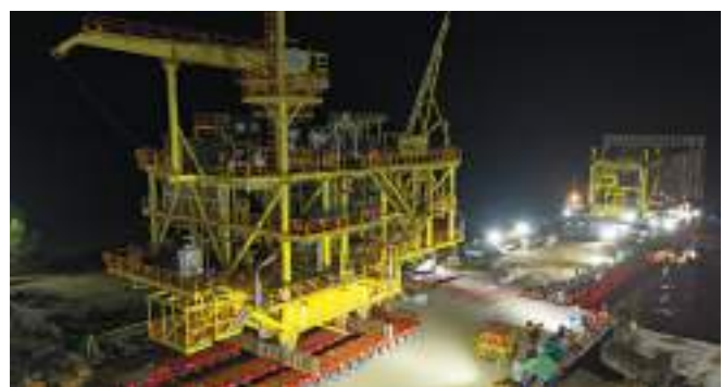
Salbiah wellhead platform load-out
