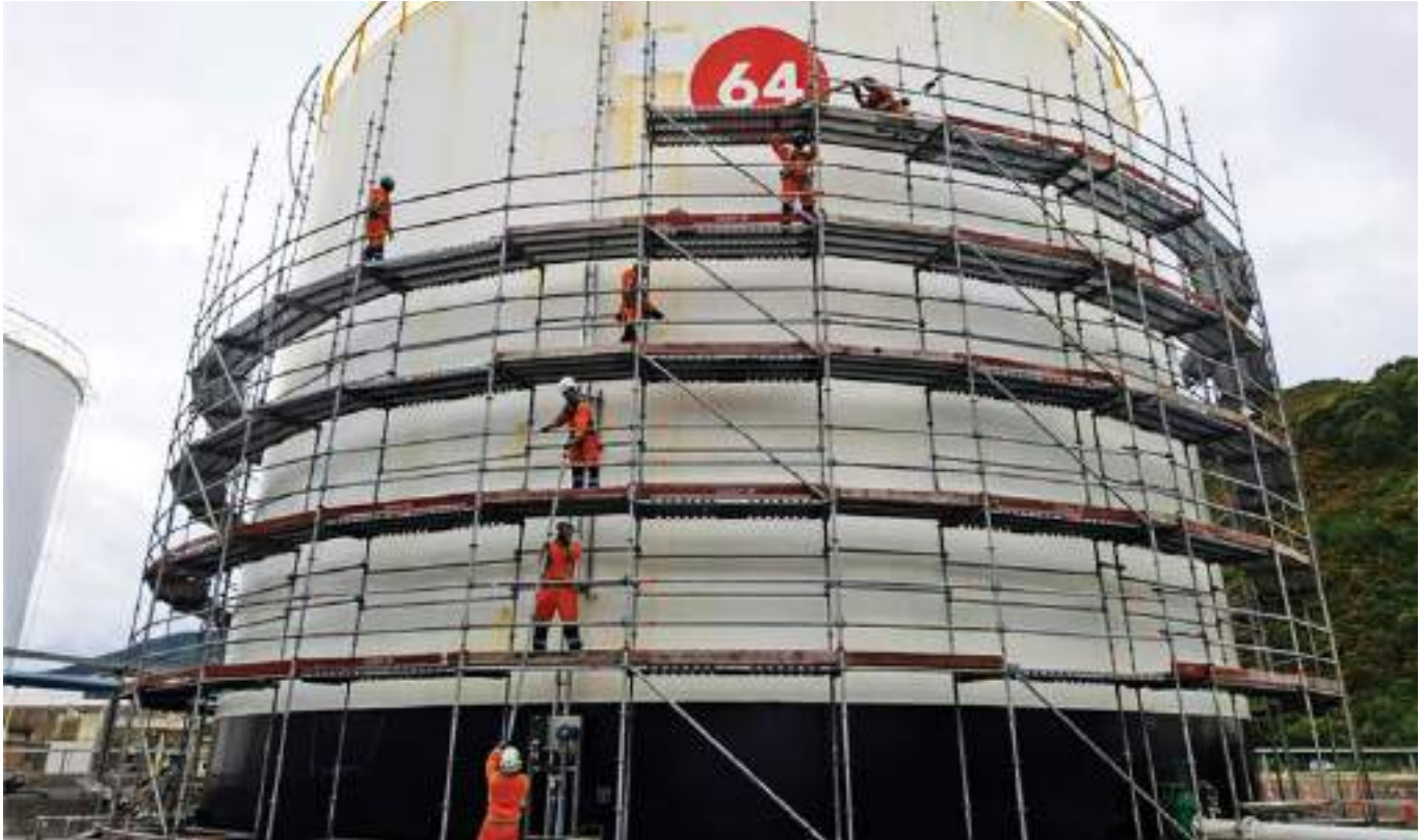
A scaffolding audit was conducted at our Fonterra Hawera project site in New Zealand as part of the mechanisms implemented to ensure conformity with safety procedures
