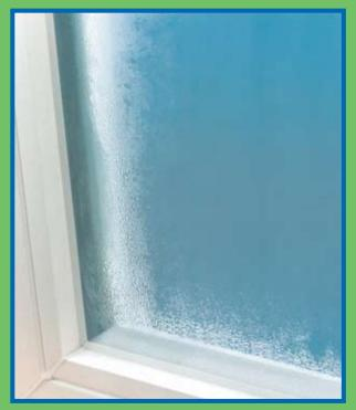
**Less-metal Spacer** Mid-performance spacer systems that still contain metal improve condensation resistance.
