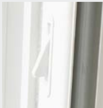
Optional sash vents limit the opening of the bottom sash.
