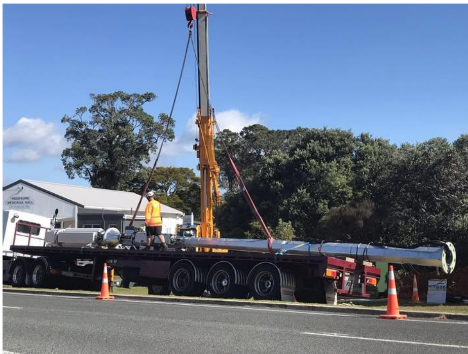
Arrival of cell tower for installation in Tutukaka (27 March 2024)
