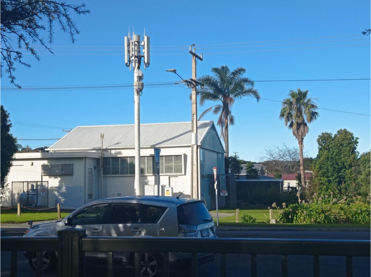
4G-5G (macro-cell) mobile tower only about 40 metres from the boundary fence of Onerahi Primary (Whangārei) – photo by the author
