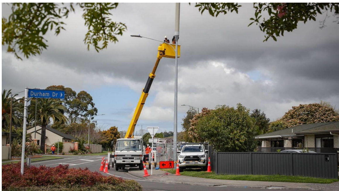
Erection of controversial cell tower in Havelock North (5 October 2021) NZ Herald Picture
