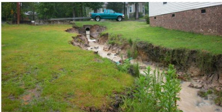
Figure 2-19: Bank erosion
