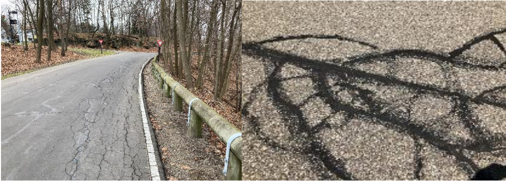
Figure 2-7: Pavement and shoulder alligator cracking
