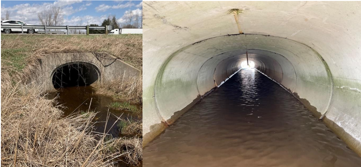
Figure 2-30: Concrete barrel culvert
