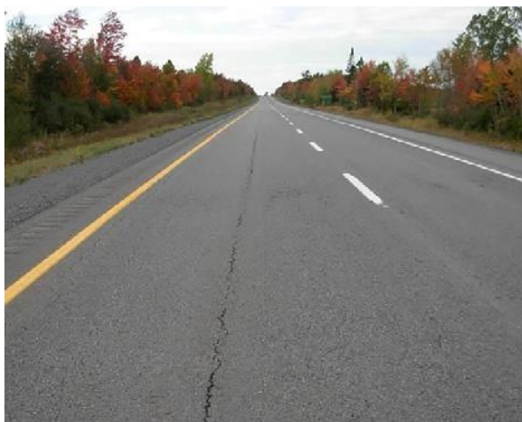
Figure 2-6: Longitudinal cracking
