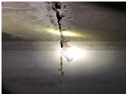
Figure 2-32: Spalling within a box culvert
