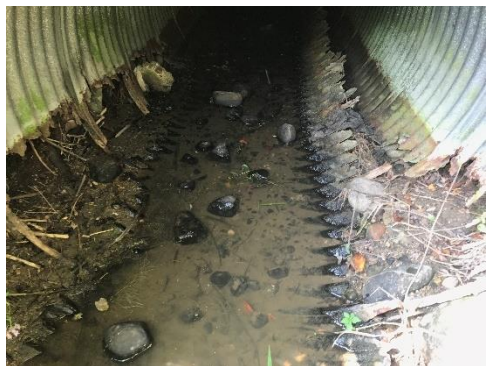
Figure 2-36: Abrasion wearing away corrugated metal pipe corrugations
