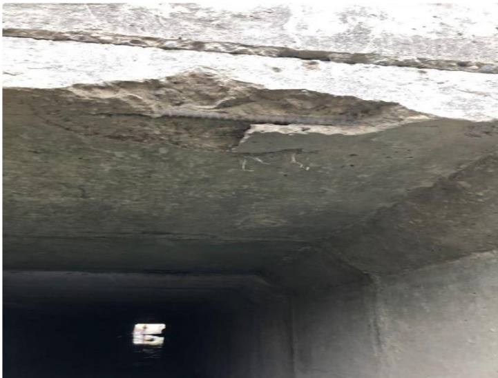
Figure 2-25: Spalled concrete at headwall
