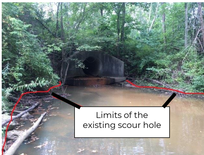
Figure 2-27: Perched outlet with large scour hole
