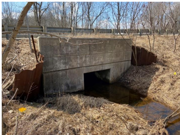
Figure 2-24: Concrete headwall and metal sheet pile wingwalls
