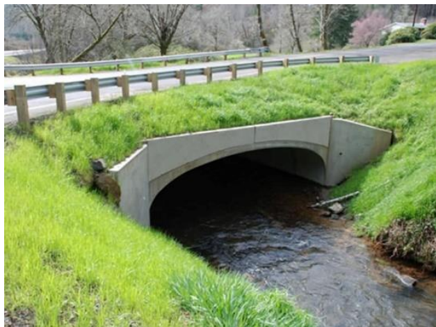
Figure 2-24: Concrete headwall and metal sheet pile wingwalls
