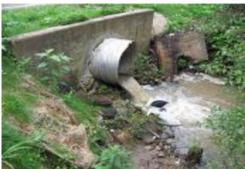
Figure 2-16: Vertical alignment distress; may have progressing washout due to high flow
