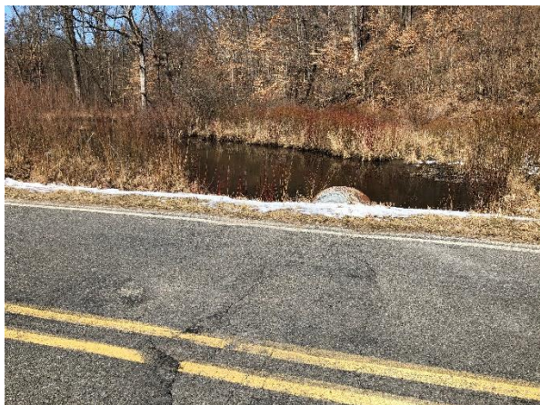
Figure 2-5: Transverse cracking of pavement above culvert
