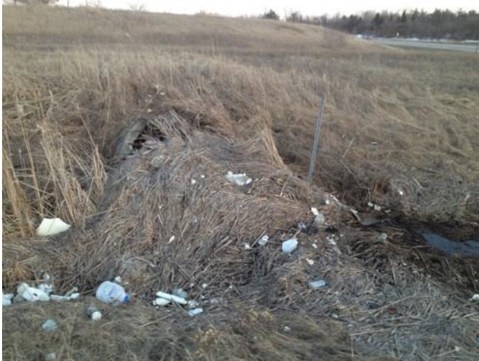
Figure 2-17: Blocked inlet
