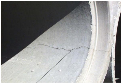
Figure 2-31: Longitudinal crack within a concrete barrel
