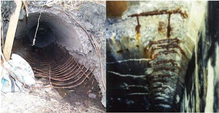
Figure 2-33: Concrete barrel deterioration
