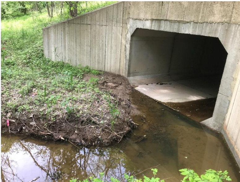
Figure 2-13: Stream channel poor horizontal alignment
