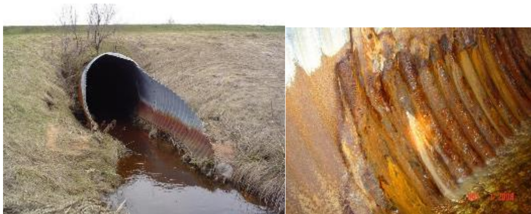
Figure 2-35: Loss of protective coatings contributing to corrosion
