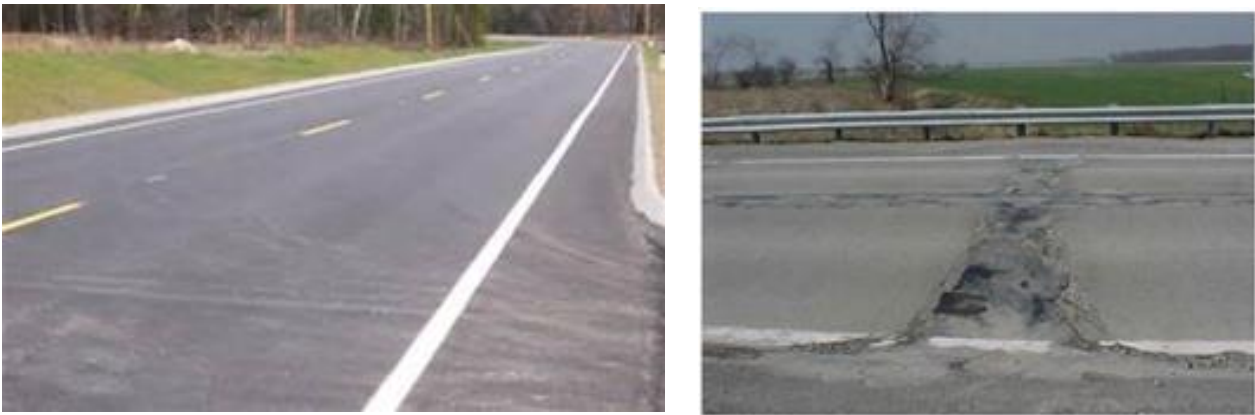
Figure 2-3: Approach roadway, without observable distress (left), clear distress over culvert (right)
