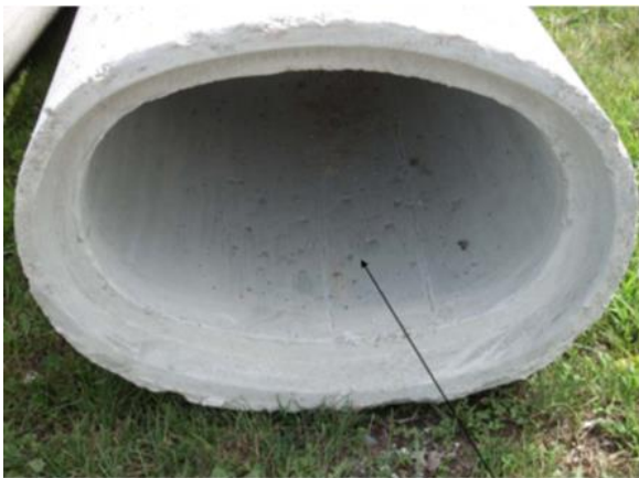
Figure 2-37: Elliptical concrete barrel
