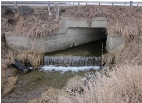
Figure 2-16: Vertical alignment distress; may have progressing washout due to high flow
