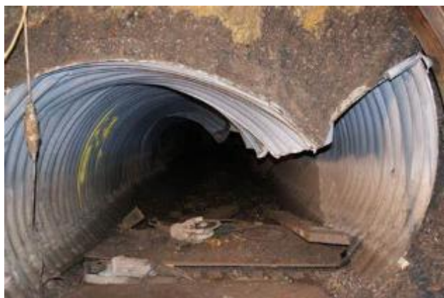
Figure 2-29: Loss of vertical alignment in a corrugated metal culvert
