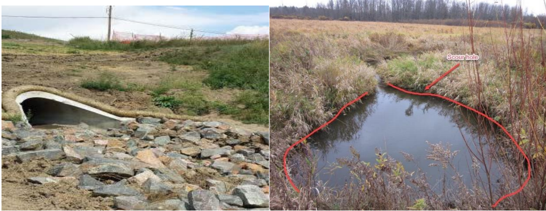
Figure 2-20: No scour (left), scour hole (right)
