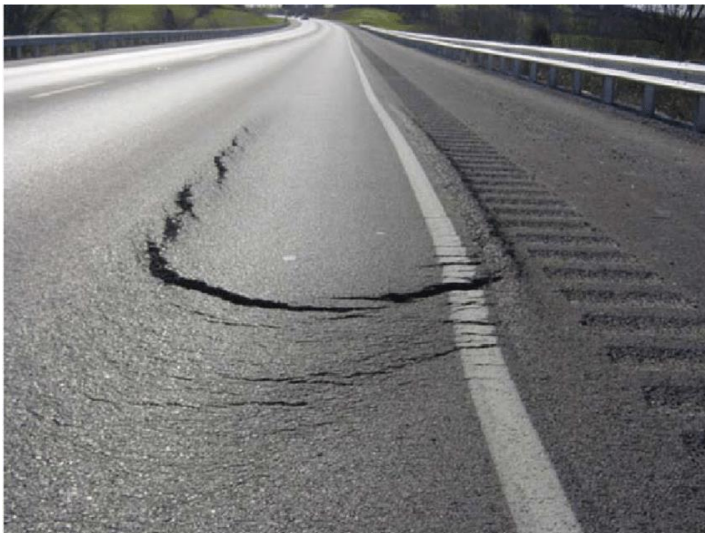
Figure 2-8: Slippage cracking
