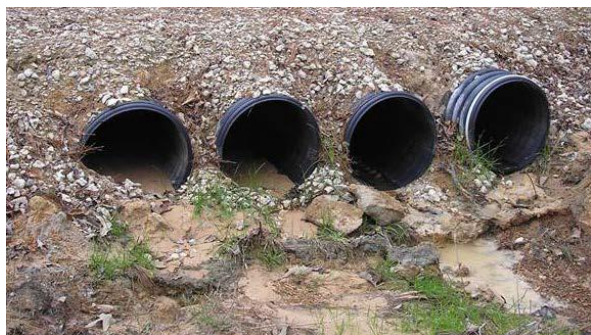
Figure 2-11: Culvert erosion—early-stage gully/rill erosion between the culverts
