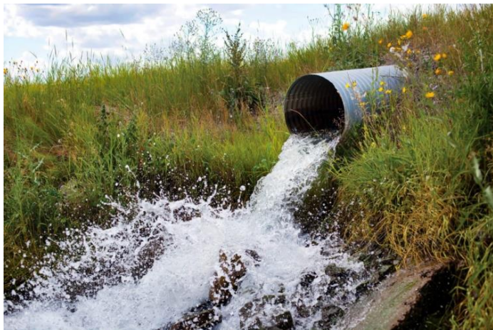
Figure 2-21: Projecting or perched outlet
