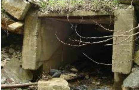
Figure 2-15: Vertical alignment issue leading to stream degradation
