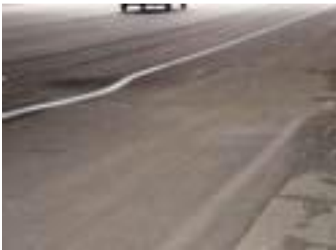
Figure 2-4: Pavement and shoulder issues above culverts
