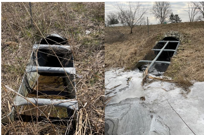
Figure 2-22: Sloped metal end sections
