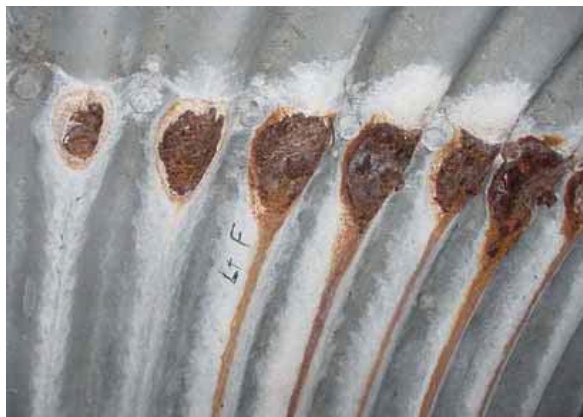
Figure 2-34: Corrosion of a metal culvert
