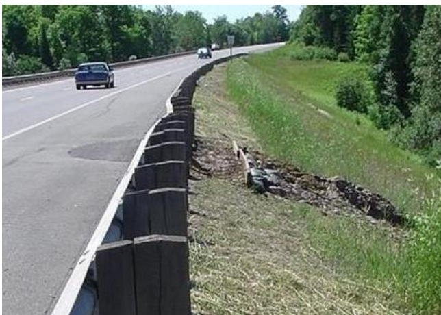
Figure 2-10: Example of embankment issues due to piping (left) or erosion (right)
