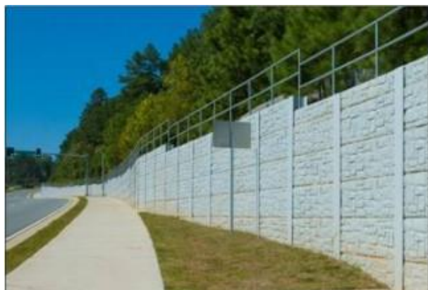
Figure 3-29: Soldier pile wall with precast lagging (note: anchors not shown)
