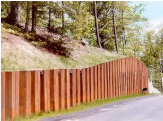
Figure 3-26: Typical metal bin wall
