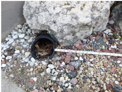
Figure 3-42: Drainage outlet is partially clogged with leaves and debris
