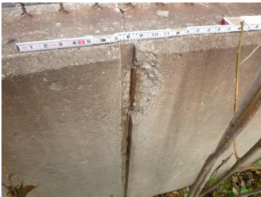
Figure 3-11: Concrete spall with corroded reinforcing
