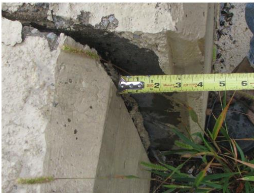
Figure 3-35: Wall displacement
