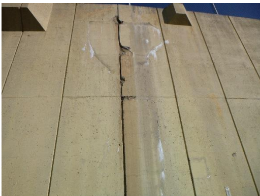
Figure 3-15: Efflorescence accumulation
