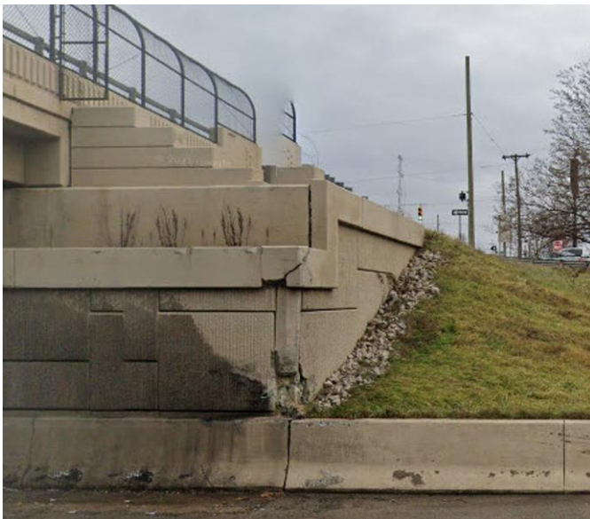
Figure 3-17: Impact damage
