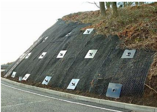
Figure 3-31: Typical soil nail wall
