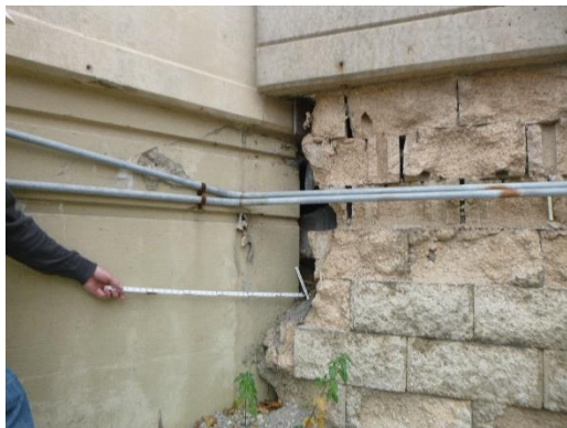
Figure 3-23: Masonry breakdown
