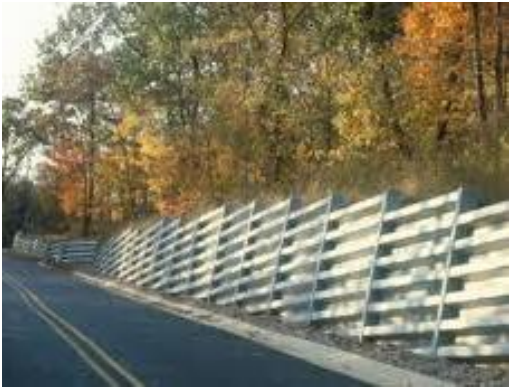
Figure 3-26: Typical metal bin wall
