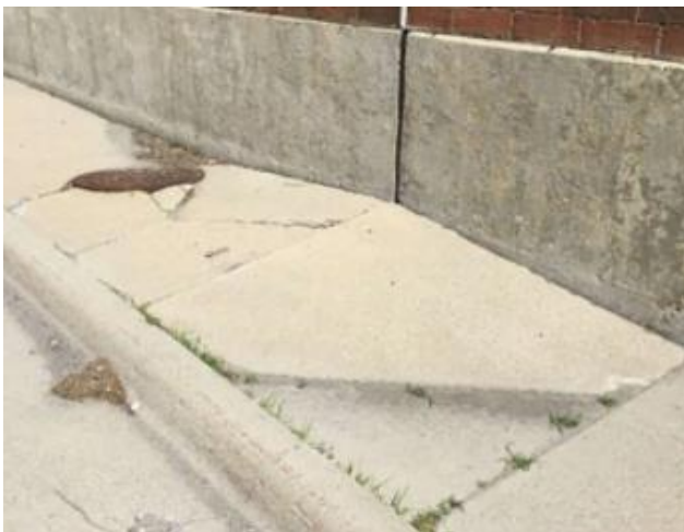
Figure 3-41: Wall settlement
