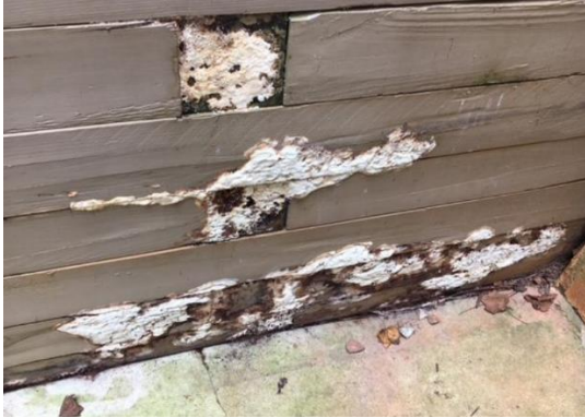
Figure 3-20: Timber lagging splitting
