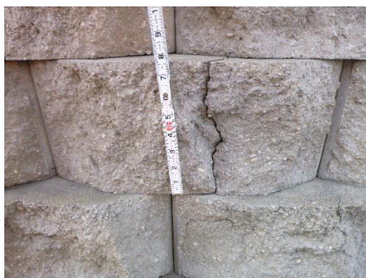
Figure 3-22: Vertical split in modular block
