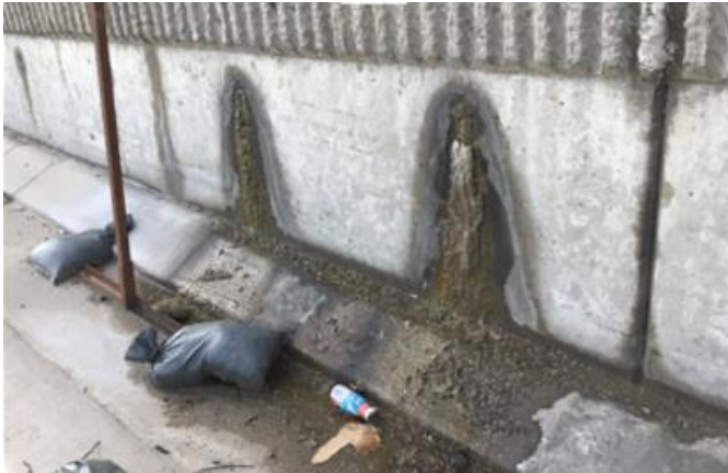
Figure 3-16: Weep holes/wall drainage
