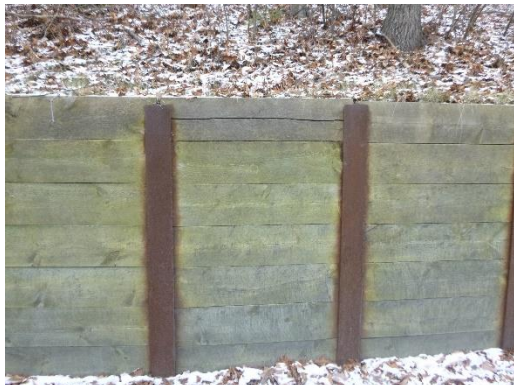
Figure 3-21: Timber lagging is split along top
