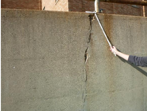
Figure 3-12: Spalled and delaminated concrete
