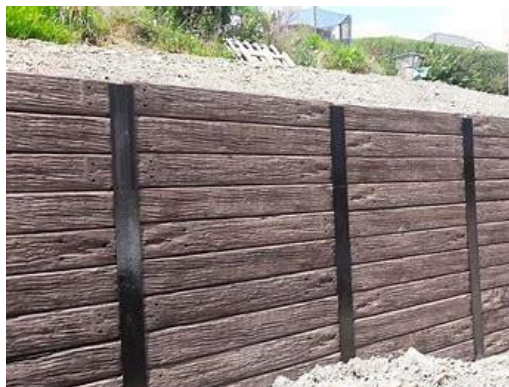
Figure 3-37: Vertical support steel
