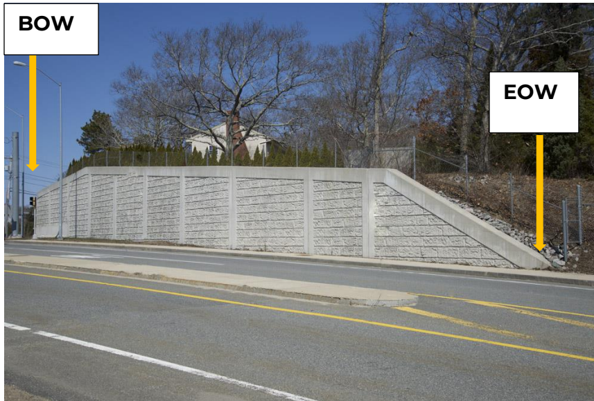
Figure 3-8: Typical wall facing inspection limits
