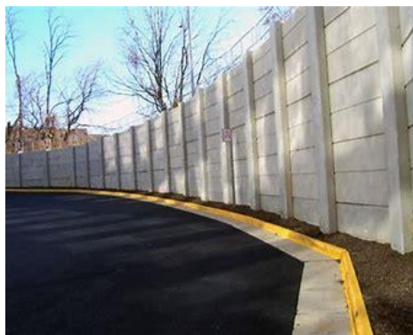
Figure 3-38: Vertical support concrete
