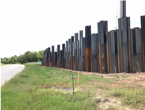
Figure 3-28: Steel protective coating missing
