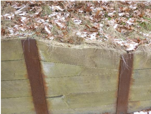
Figure 3-20: Timber lagging splitting
