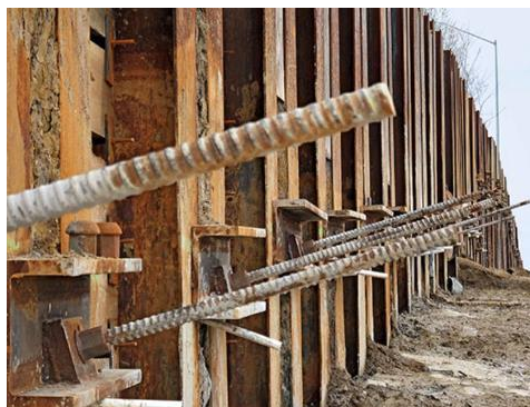
Figure 3-36: Wall anchor
