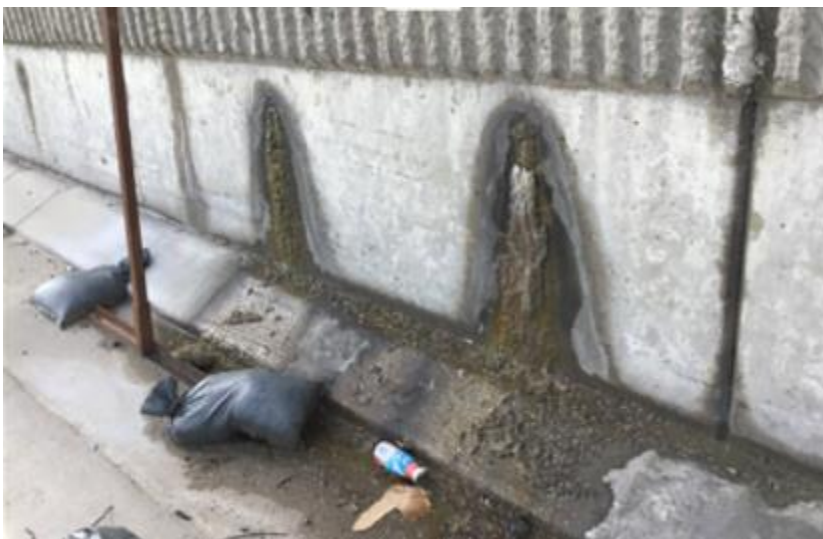
Figure 3-13: Retaining wall concrete abrasion
