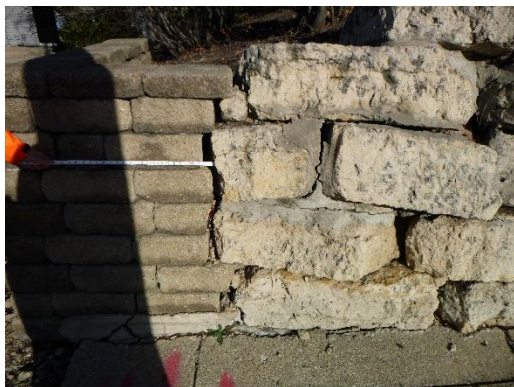
Figure 3-24: Wall misalignment
