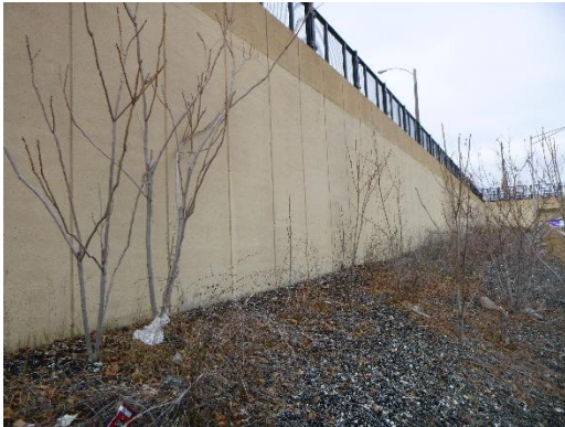
Figure 3-14: Semi-protective concrete protective coating
