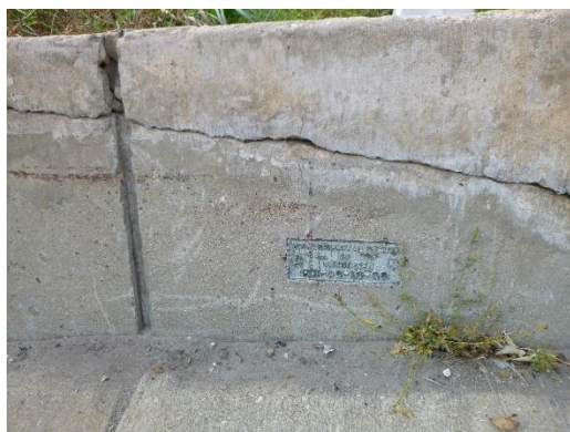
Figure 3-9: Horizontal structural cracking
