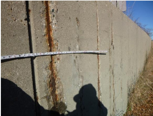
Figure 3-10: Corroded wall reinforcing
