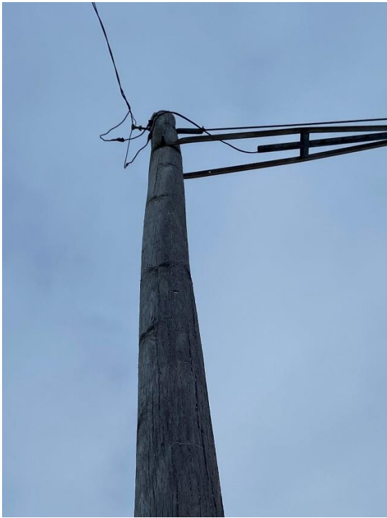
Figure 5-10: Minor crook in wood pole
