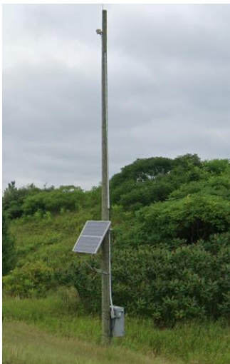
Figure 5-3: Embedded wood pole supporting ITS infrastructure
