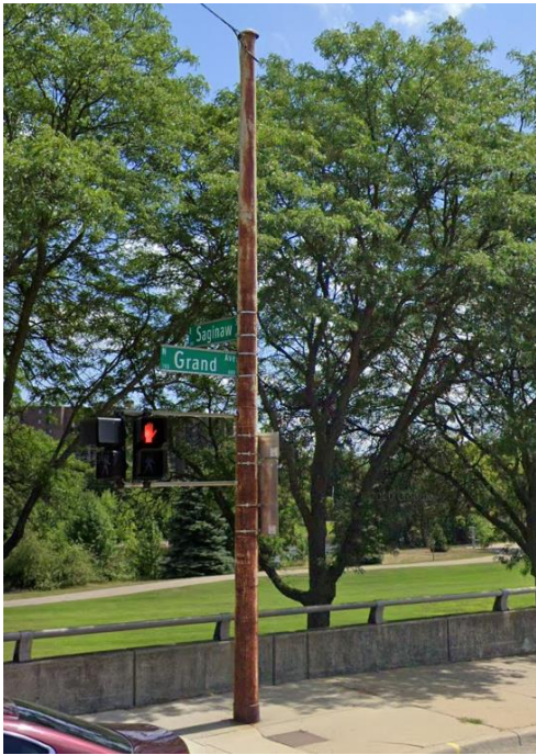
Figure 5-14: Embedded Pole with heavy corrosion, concrete sidewalk covering embedment material
