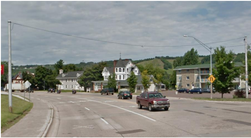
Figure 5-2: Embedded steel poles with single span configuration
