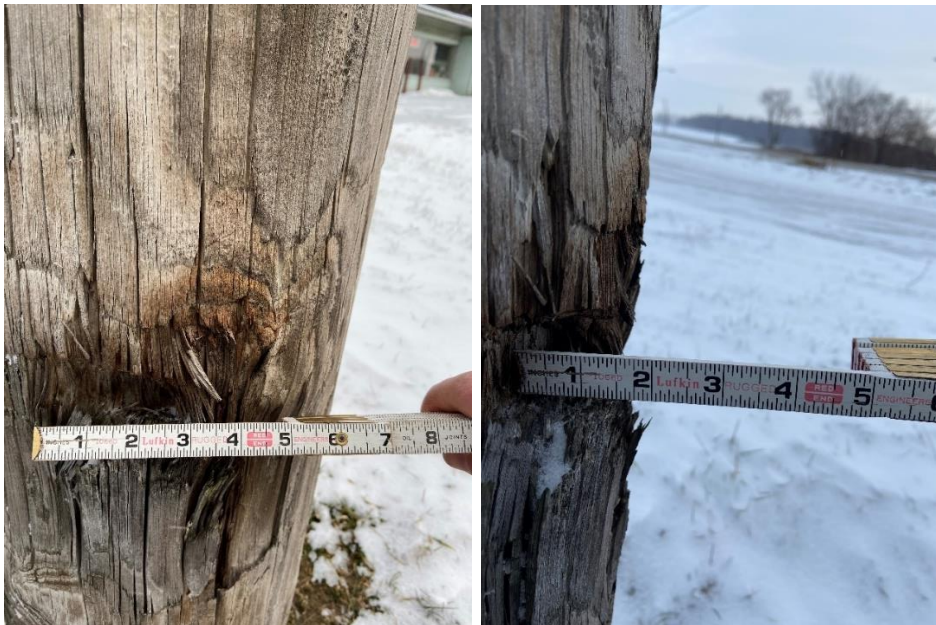
Figure 5-13: Measuring impact damage
