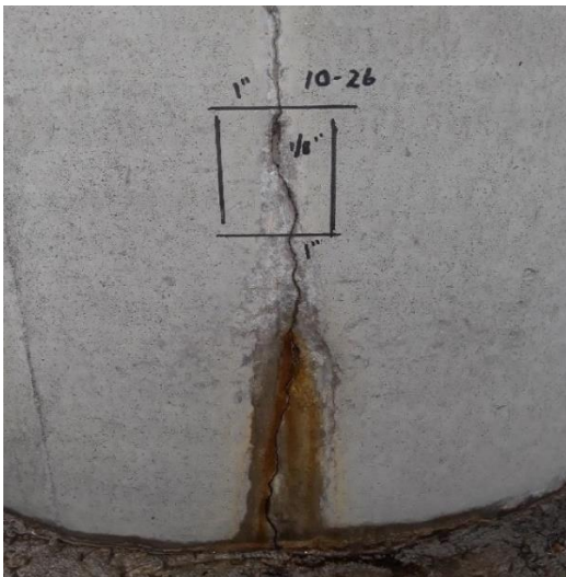
Figure 6-5: Crack with rusted rebar water leakage
