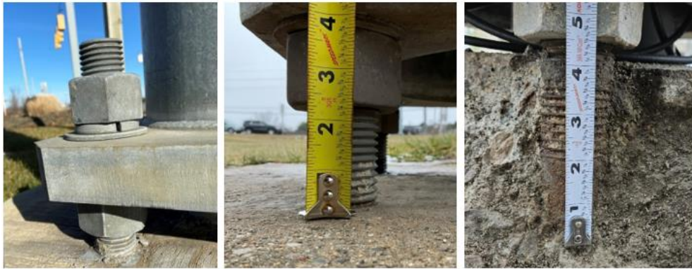
Figure 7-8: Fully compressed lock washer (left), Standoff measurement for a sound foundation (middle) and standoff measurement with foundation concrete deterioration (right)
