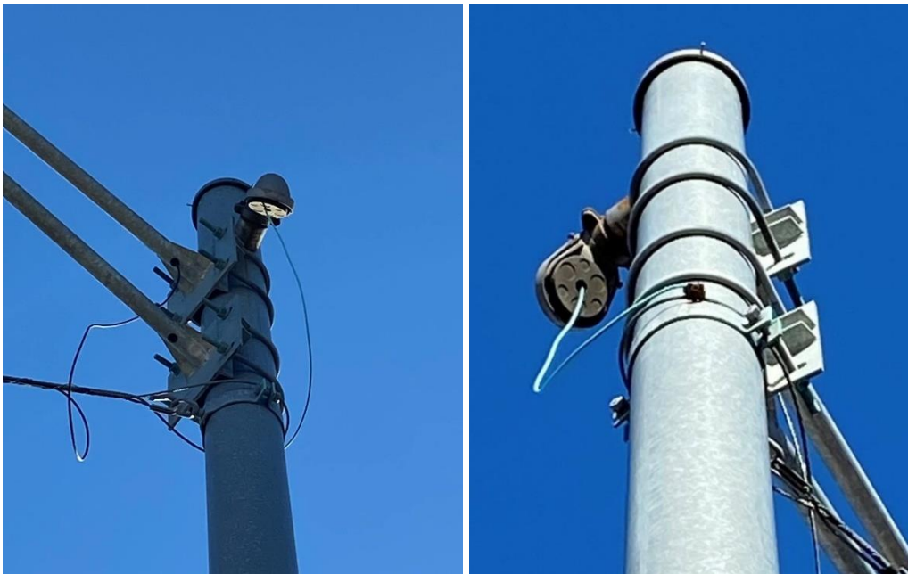
Figure 7-13: Steel strain pole bracket assembly connections for luminaire arms
