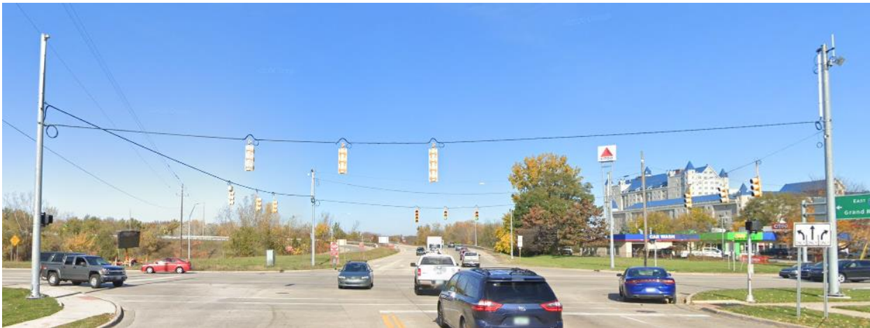
Figure 7-4: Steel strain poles with single diagonal span configuration
