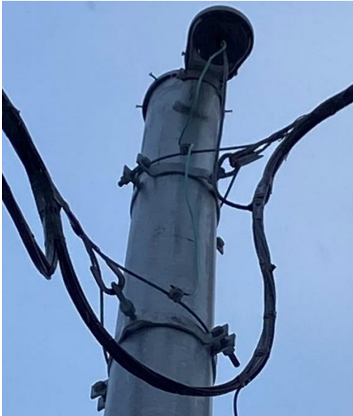
Figure 7-13: Steel strain pole bracket assembly connections for luminaire arms
