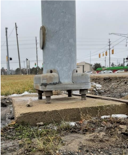
Figure 7-9: Steel strain pole foundation with excess standoff distance and nut covers
