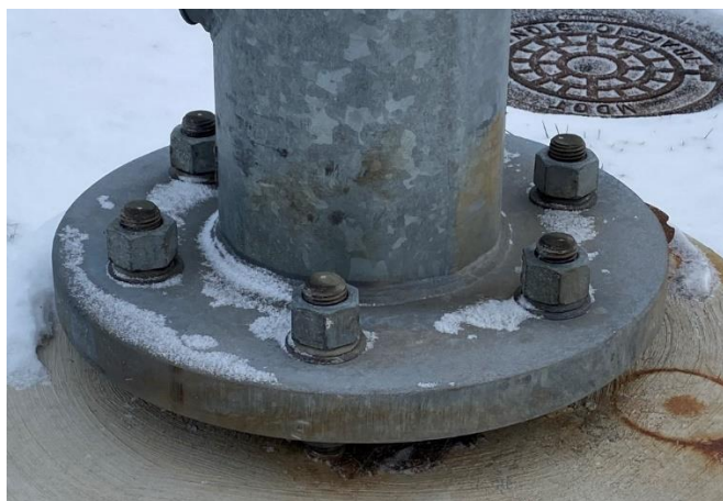
Figure 7-10: Steel strain pole base plate with six anchor bolts
