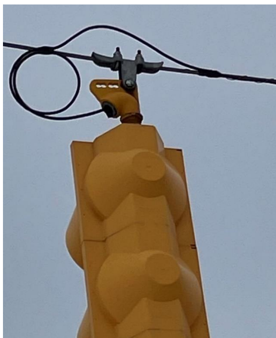
Figure 7-17: Span wire hanger
