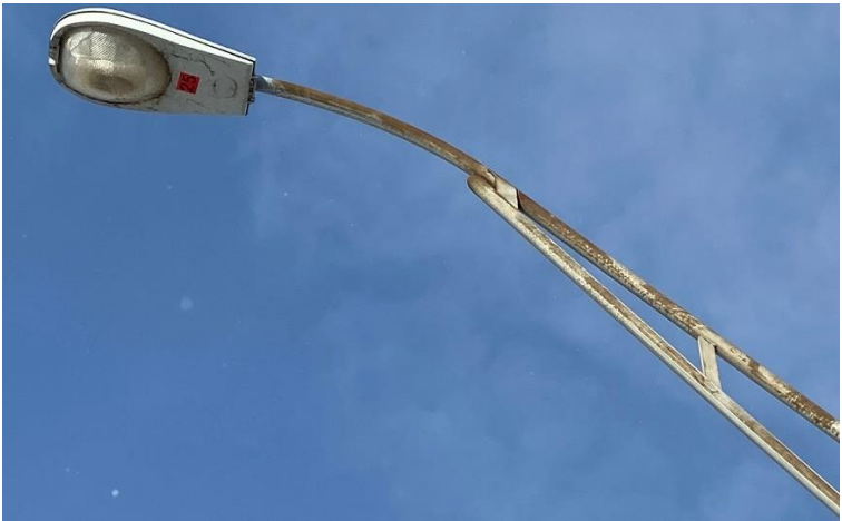
Figure 7-18: Luminaire and luminaire truss arm
