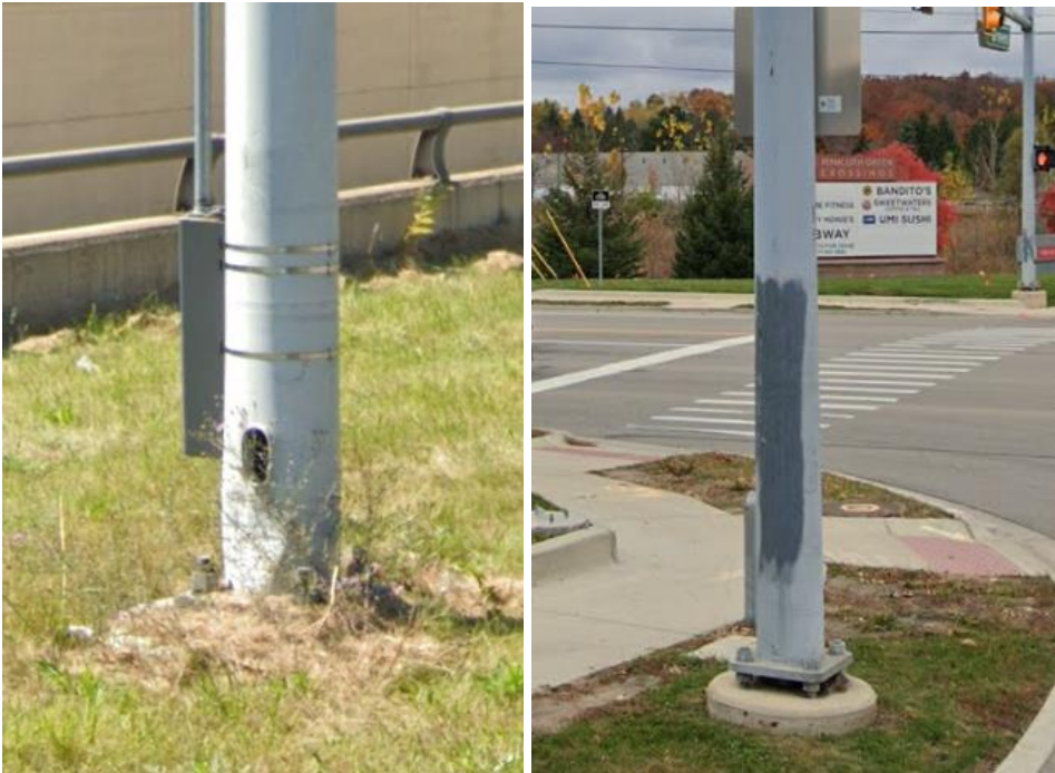
Figure 7-11: Impact damage and missing hand hole cover (left) and graffiti/coatings repair (right)
