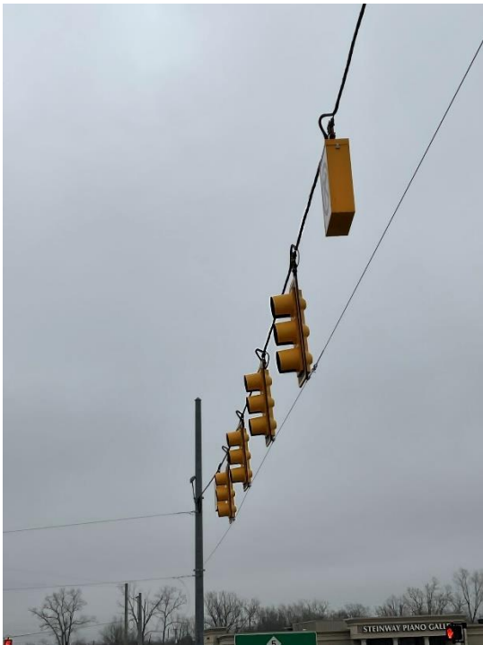
Figure 7-14: Steel strain pole span wire supporting signals and sign
