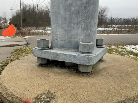
Figure 7-9: Steel strain pole foundation with excess standoff distance and nut covers
