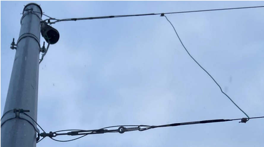
Figure 7-15: Span wire assemblies attached to steel strain pole band clamps
