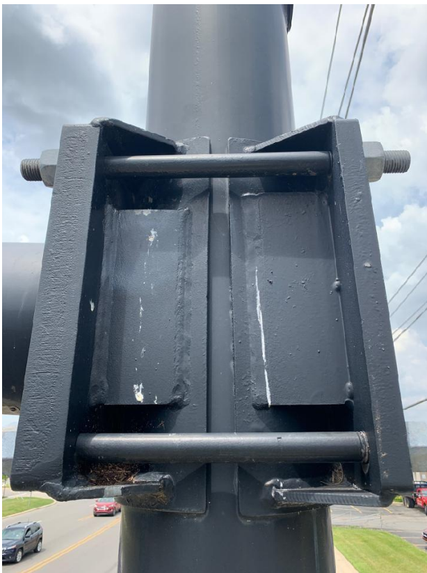
Figure 9-13: Mast arm vertical structure connection, note missing vertical weld on gusset plate
