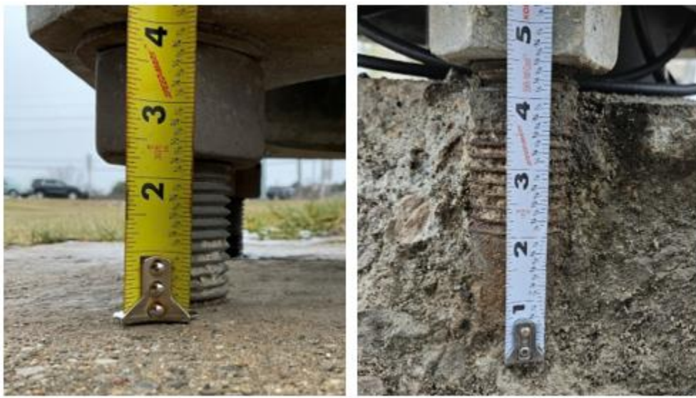
Figure 9-6: Standoff measurement for a sound foundation (left) and standoff measurement with foundation concrete deterioration (right)
