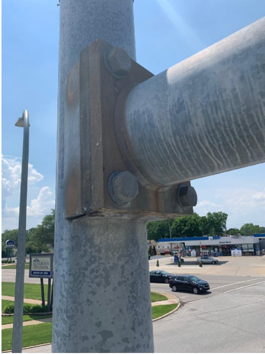
Figure 9-13: Mast arm vertical structure connection, note missing vertical weld on gusset plate
