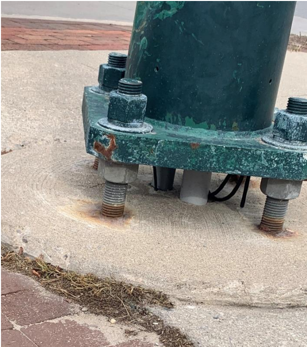
Figure 9-8: Four anchor bolt foundation with excessive standoff distance and corrosion
