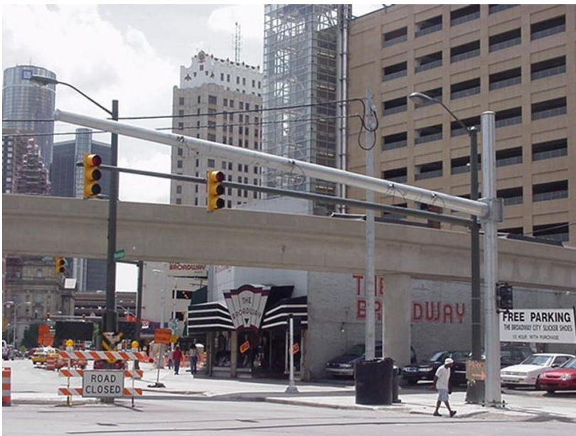
Figure 9-1: MDOT Category I Mast Arm, note previous design in background before removal
