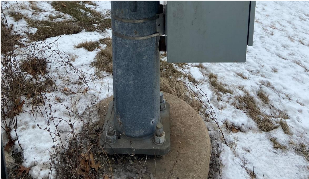
Figure 9-9: Mast arm base plate with four anchor bolts
