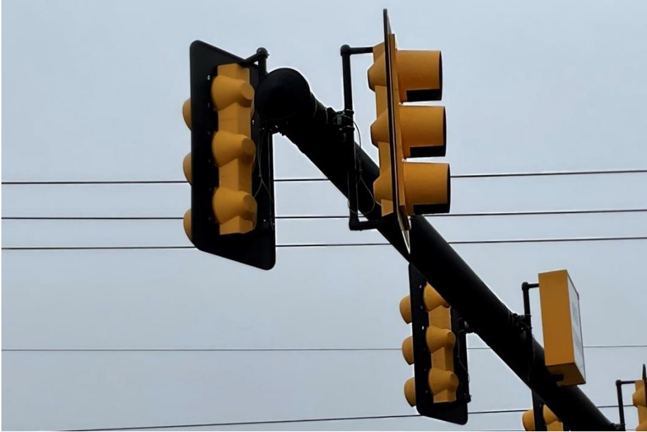
Figure 9-16: Mast arm signal and sign attachment connections
